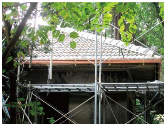
裝設銅管落水頭與天溝
